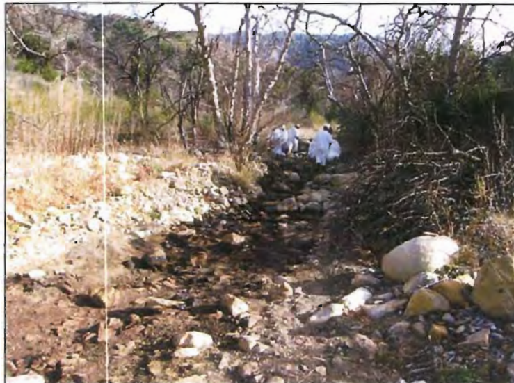
Picture 1- Surface flows in Segment 5 were not present in channel by the time the cleanup got underway. Spilled oil became stranded on/in streambed as natural stream flows diminished. ACTI work crews were clearing debris from low-flow channel to facilitate cleanup and to prevent underflow dams from clogging in case of rain. (pic id: 228_kw, pic date: 02/06/07)
