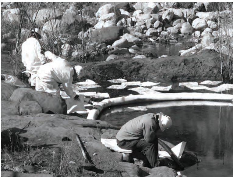
Rocks along the creek bank are covered in sludge while globs of oil float downstream. Workers in hazmat suits use flotation devices, absorbent pads, and a suction hose to remove the oil from the creek.
